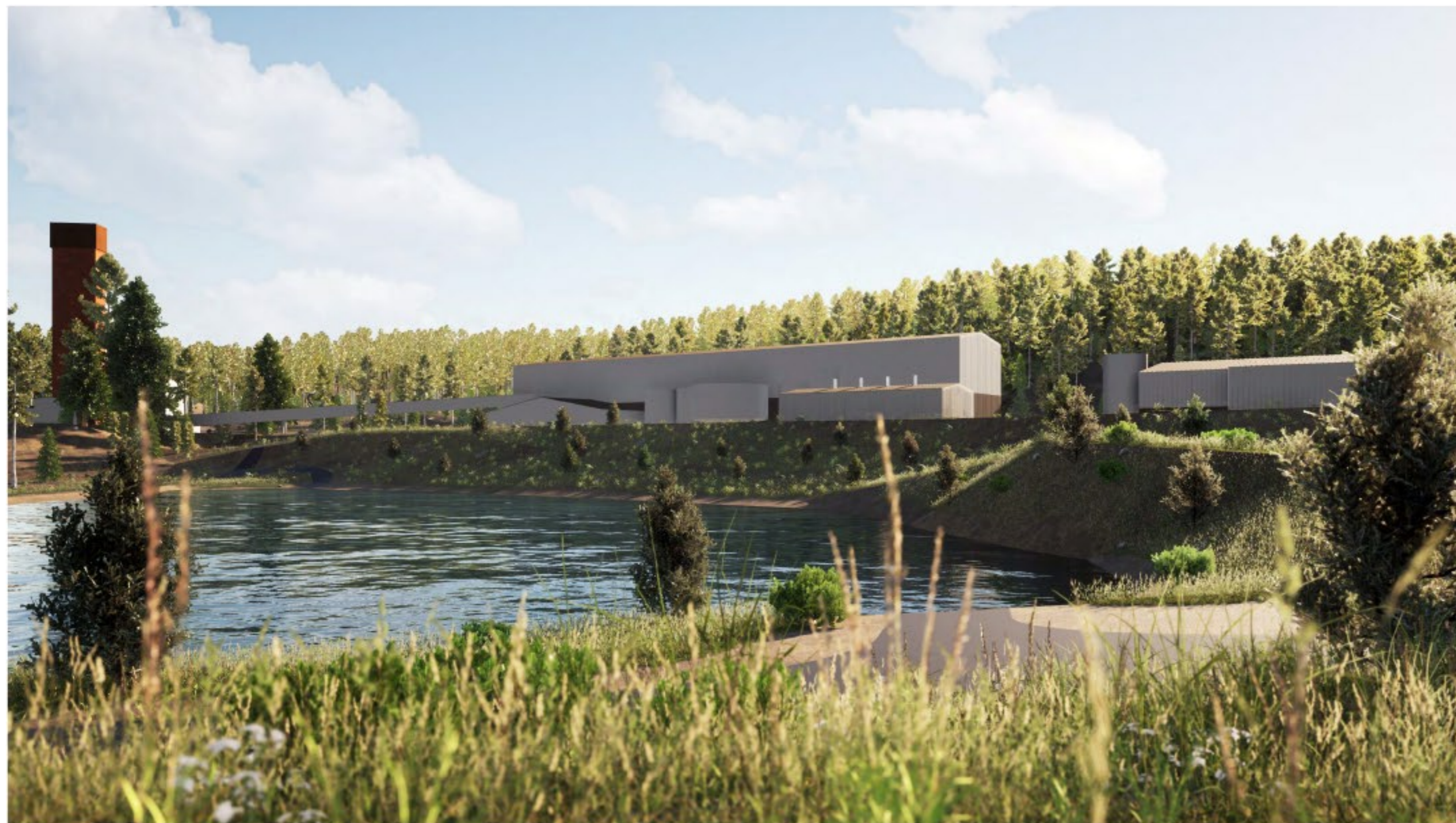
2 PROCESSING PLANT (WEST)
