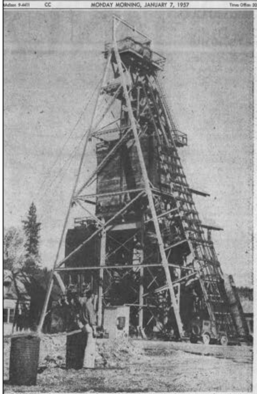
DESERTED—Increased costs forced this Idaho Maryland mine near Grass Valley to close. Jack Clark, superintendent, stands before the deserted shaft of the mine.
